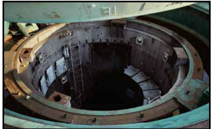
Launch Silos 40 Total
